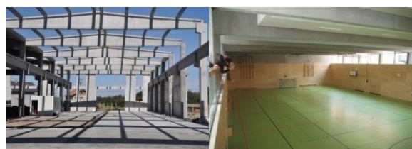
Fig. 4 Prefabricated hall made from reinforced concrete “sandwich” elements
