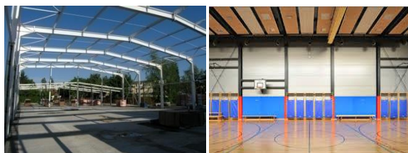
Fig. 2 Steel hall made with “sandwich” panels
