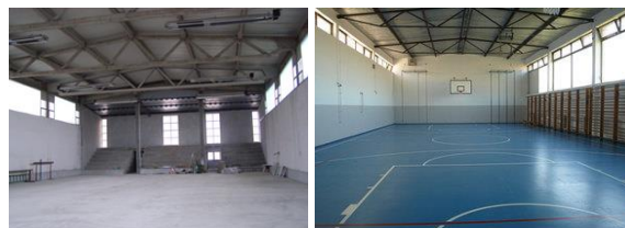
Fig.3 Hall made of clay blocks with steel roof
