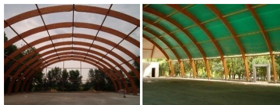
Fig. 1 Ballon hall with wooden structure
