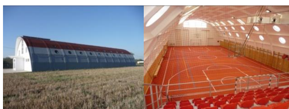
Fig.5 Prefabricated hall made from ferrocement sandwich elements
